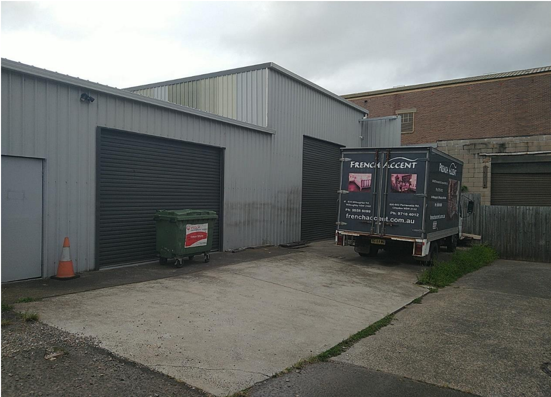
Photo 1: Rear laneway access
