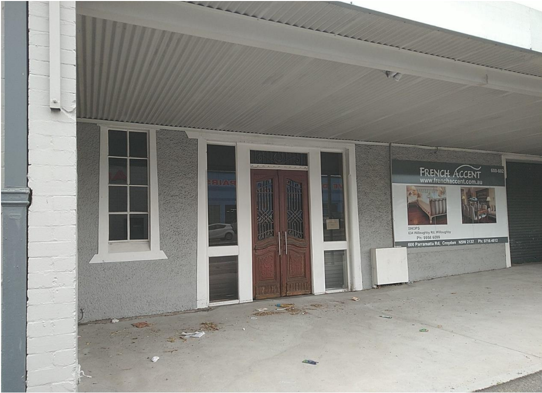
Photo 3: Shop front along Parramatta road
