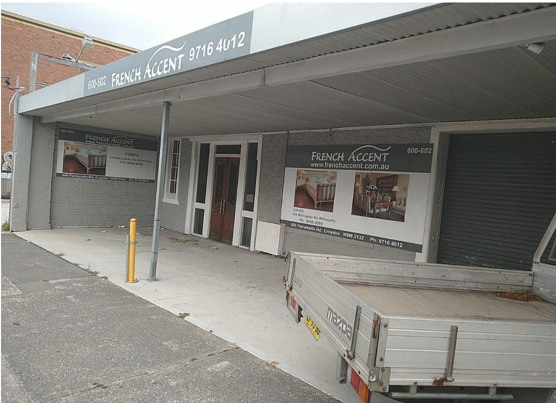
Photo 2: Shop front along Parramatta road 2
